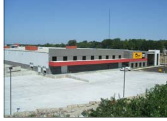
Concrete Parking Lot Award Dean Machinery 87th & I-435, KCMO
