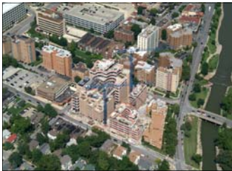
High Rise Concrete Award West Edge Office & Hotel Roanoke Pkwy, KCMO
