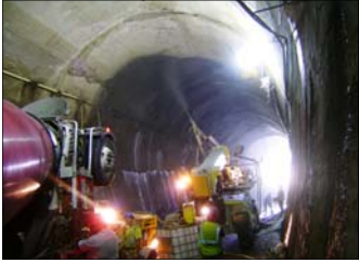
Concrete Restoration Award Turkey Creek Tunnel Kansas City, KS
