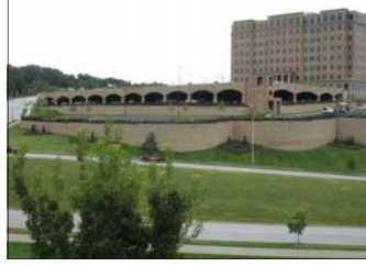
Parking Garage Award Briarcliff Village Office Parking Garage Kansas City, MO
