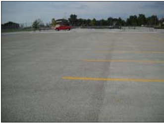
Pervious Concrete Oregon Trail Parking Lot Olathe, KS
