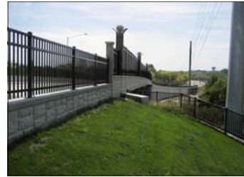
Bridge MoDot Pryor Road Bridge Lee's Summit, MO
