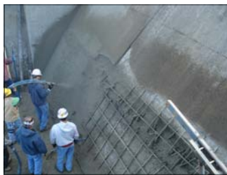
Concrete Restoration Lake Olathe Dam Stabilization Olathe, KS
