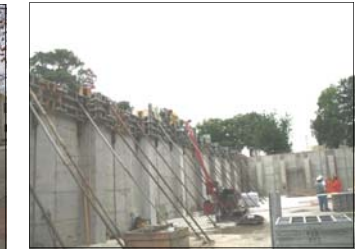
Structural Concrete UMKC Miller Nichols Library Addition, Kansas City, MO
