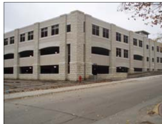
Parking Garage K-State Parking Garage Manhattan, KS
