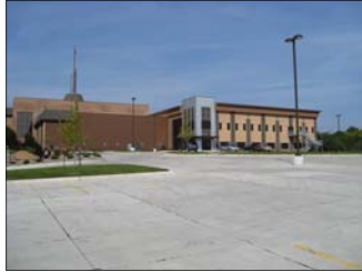
Concrete Parking Lot Evangel Temple Kansas City, MO
