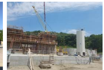
Water Treatment Plant Parkville Water Treatment Plant Parkville, MO
