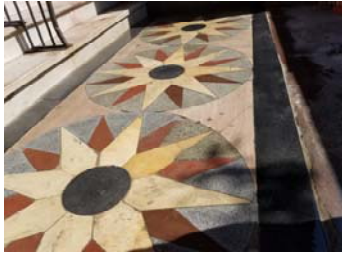
Restoration New England Mosaic Kansas City, MO
