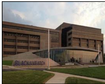
Low Rise Black & Veatch Innovation Pavilion Overland Park, KS
