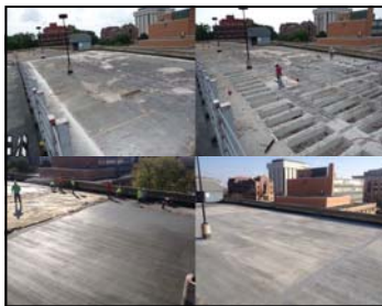
Restoration Parking Facility C - 7th & Ann Kansas City, KS
