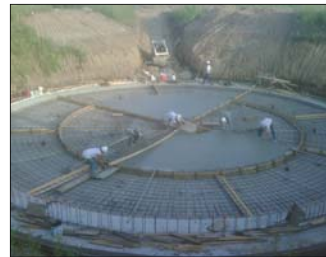
Wastewater Treatment Harrisonville Wastewater Treatment Expansion
