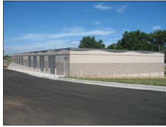
Structural Aesthetics Cerner LS-V Improvements
