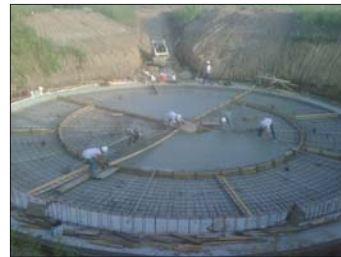
Wastewater Treatment Harrisonville Wastewater Treatment Expansion
