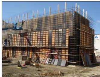
Concrete Building Bradken Gamma Ray Building
