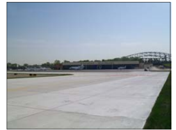
Airport Paving Wheeler Airport Runway 1/19 Safety Area
