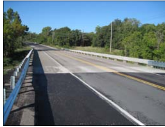
Concrete Restoration Old Hwy 56 Bridge Rehabilitation
