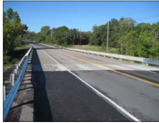
Concrete Restoration Old Hwy 56 Bridge Rehabilitation
