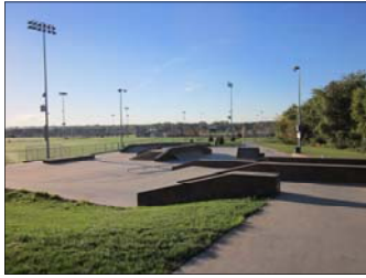
Recreation Project Overland Park, KS Skate Park
