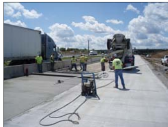
Paving DOT Hwy 350 & I-470 Paving & Bridges
