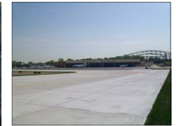
Airport Paving Wheeler Airport Runway 1/19 Safety Area
