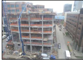
High Rise Children's Hospital East Tower Kansas City, MO
