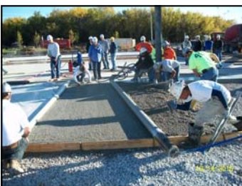
Pervious Paving Kansas BioScience Venture Accelerator Olathe, KS
