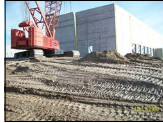
Site Cast Tilt-up EARP Distribution Center Edwardsville, KS
