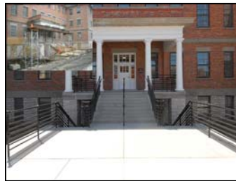
Concrete Restoration Building 465, Ft. Leavenworth Leavenworth, KS
