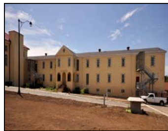
Concrete Renovation Fort Leavenworth Historical Buildings 466/467 Leavenworth, KS
