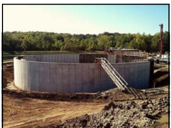
Wastewater Treatment Plant Fishing River Plant Kansas City, MO
