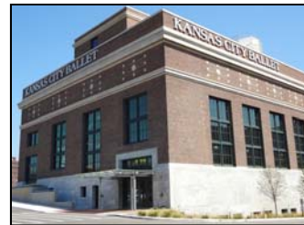
Concrete Restoration Todd Bolender Center for Dance Kansas City, MO
