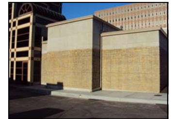
Heavy Weight Concrete Saint Luke's Linear Accelerator Kansas City, MO
