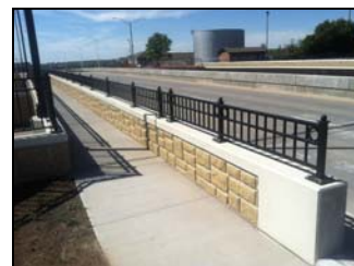
Bridge 159 th Street Bridge Overland Park, KS
